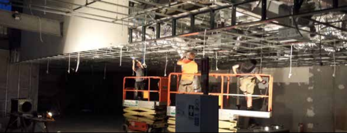
Cotton On Torquay electrical & A/C rough in.
